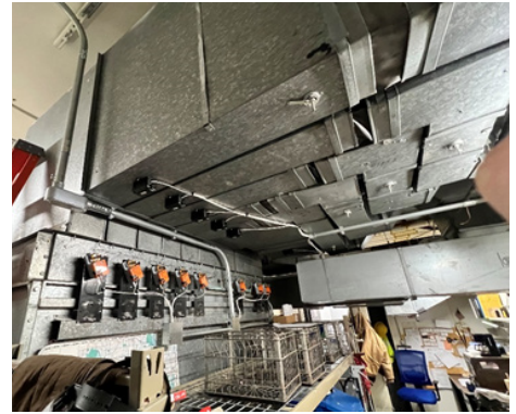
Figure 1: AHU - Multizone Dampers
