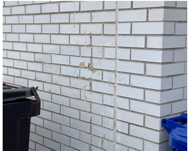
Cracked masonry at service door
