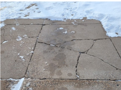
Cracked Sidewalk at Southwest Corner of Building
