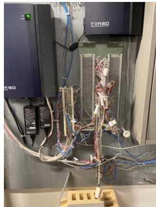
Figure 11: Voice Cabling Punch Down and Patching
