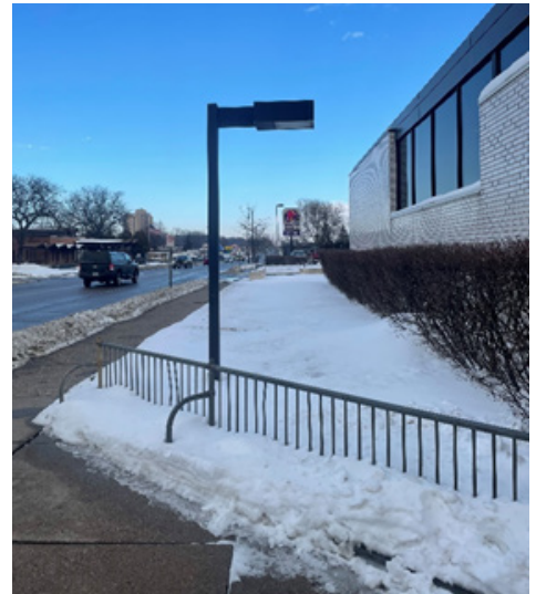
Figure 8: Short Shoebox Fixture
