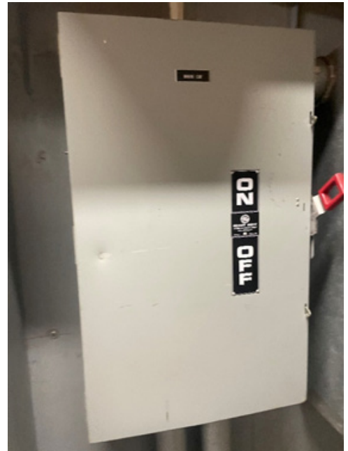
Figure 5: Main Disconnect
