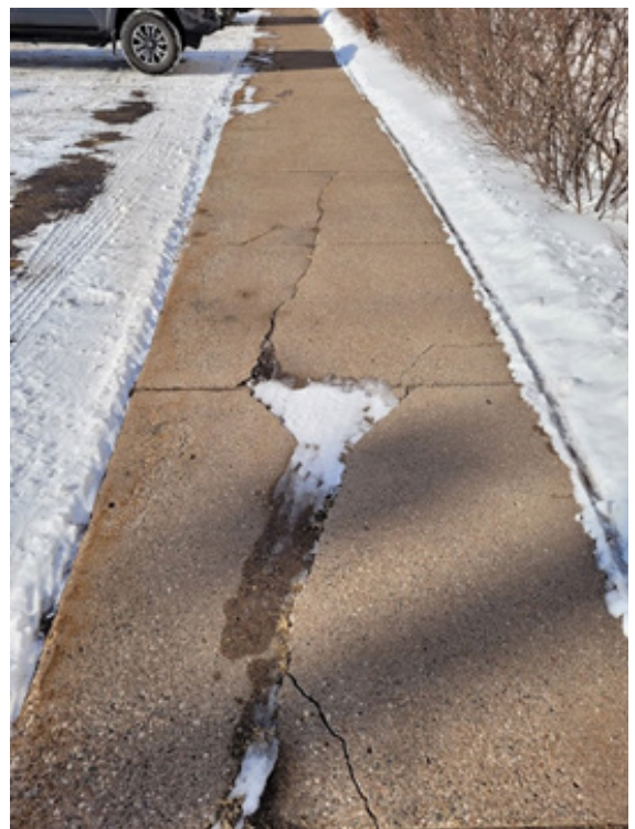
Cracked Sidewalk South of Building
