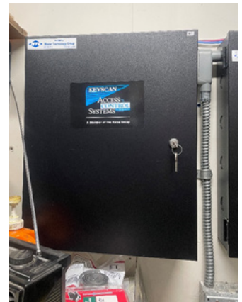
Figure 13: Access Control System
