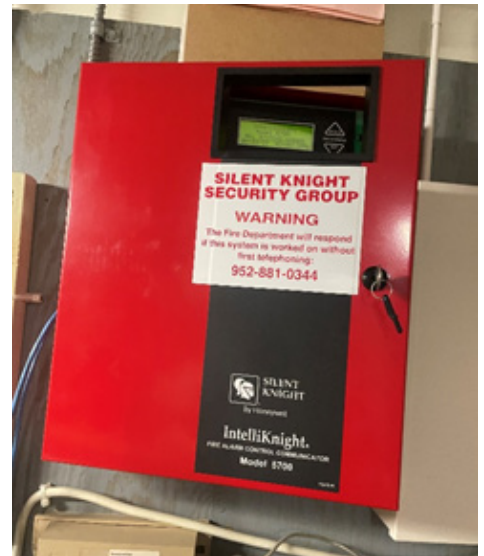
Figure 9: Fire Alarm Control Panel
