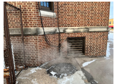
Figure 2: Boiler flue exhaust entering combustion air intake
