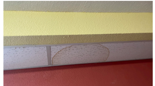
Ceiling Water Damage in Hamline Midway Coalition Office
