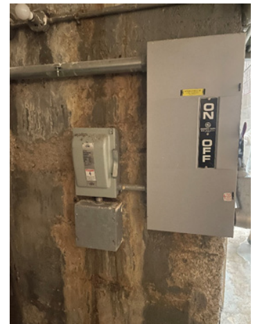
Figure 6: Main Disconnect
