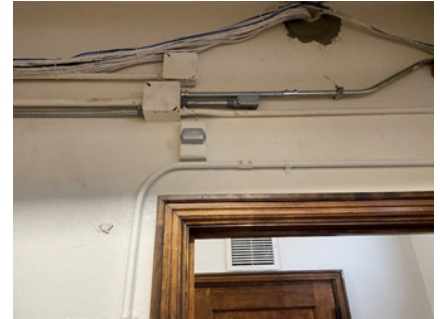
Figure 10: Exposed interior low voltage wiring
