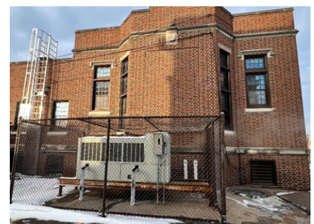
Figure 4: Air-cooled chiller
