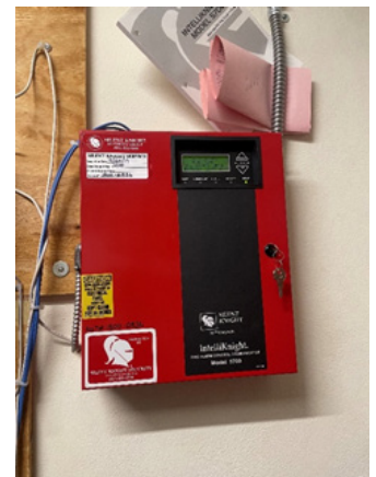
Figure 9: Fire Alarm Control Panel
