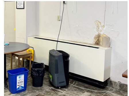
Figure 1: Unit Ventilator
