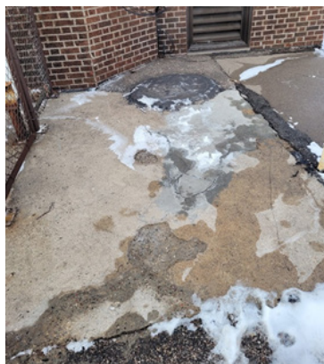
Deteriorated Concrete at Transformer
