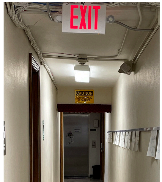
Exposed Wires at Ceiling and Low Structure in Hallway
