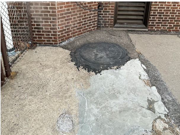
Exterior Slab degradation
