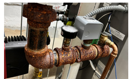
Figure 3: Boiler hydronic piping rust
