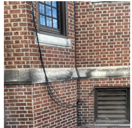
Figure 12: Exposed Exterior Low Voltage Wiring
